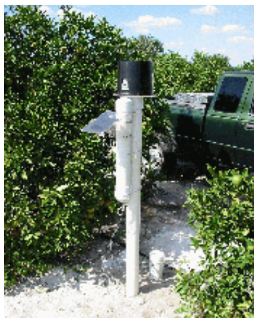
Typical installation of an instrument-sensor cluster, measuring rainfall, irrigation water pressure, watertable depth, and volumetric soil water in the citrus root zone
