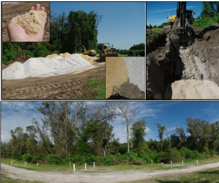
Building a denitrification wall
