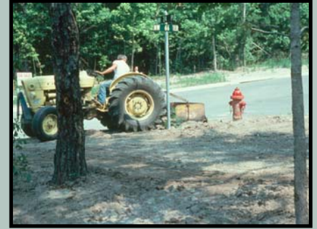
Burial of surface soil under fill material
