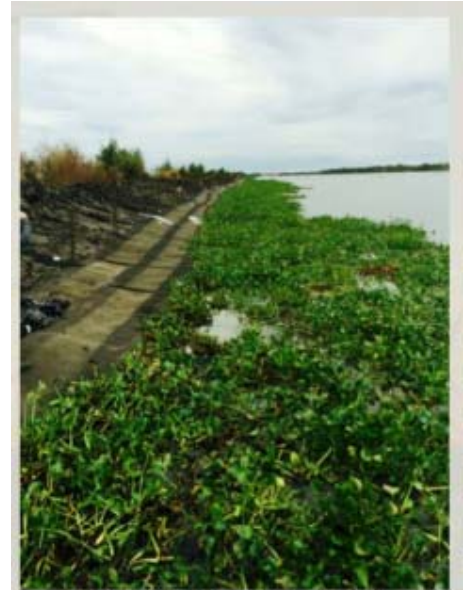
Two of four layers of EcoShield™ installed into GIWW shoreline.
