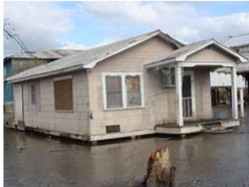
House in Isle de Jean Charles after Hurricane Gustav in 2008.
