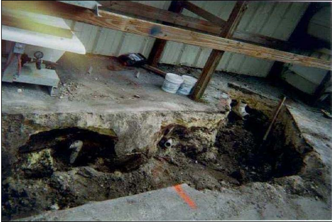
Figure 18: Excavated drains at site
