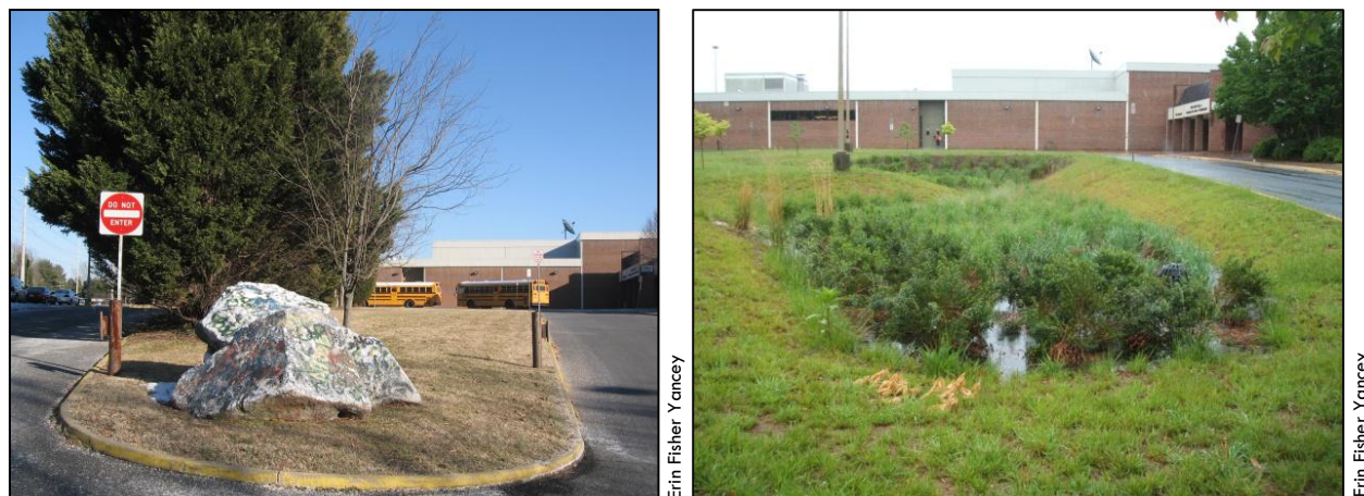
FIGURE 1. TRAFFIC ISLAND, BEFORE AND AFTER THE ADDITION OF THE BIOFILTER.
