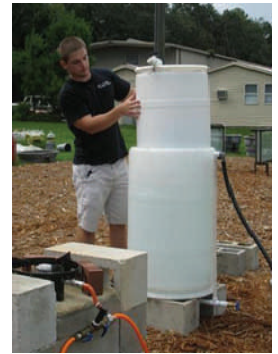
Tim Sink building an anaerobic digester for generating biogas
