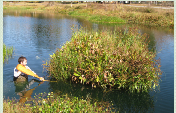
Floating Wetland Treatment System after 8 months deployment in stormwater detention pond
