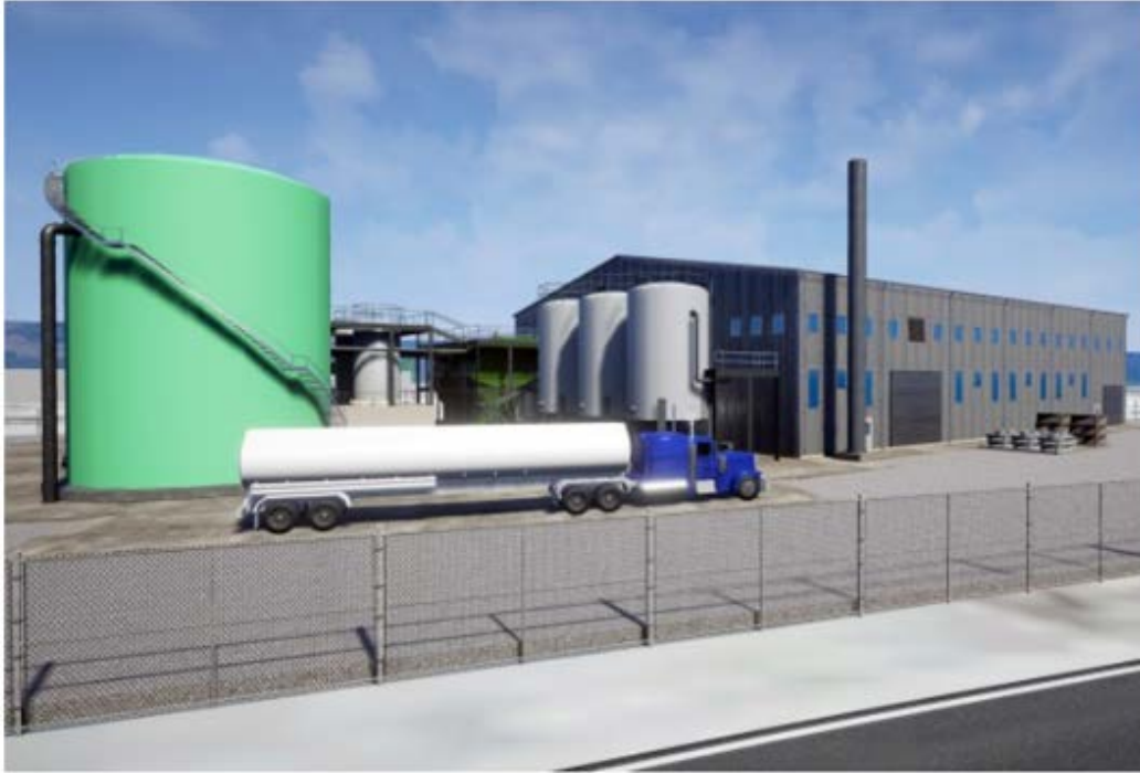
Figure 11 Mercury Treatment Facility of the Outfall 200 Mercury Treatment Facility (Huotari, 2017).
