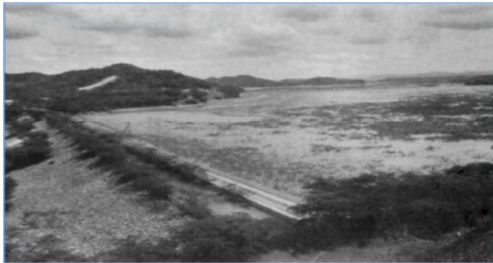
Figure 4: The fully cemented Camare irrigation reservoir in Venezuela. This reservoir filled with silt in only 15 years(Morris & Fan, 1998, p. 45).
