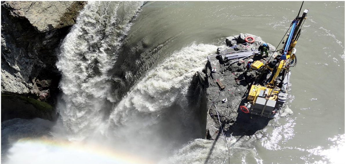
Workers prep for explosives placement on Glines Canyon Dam.
