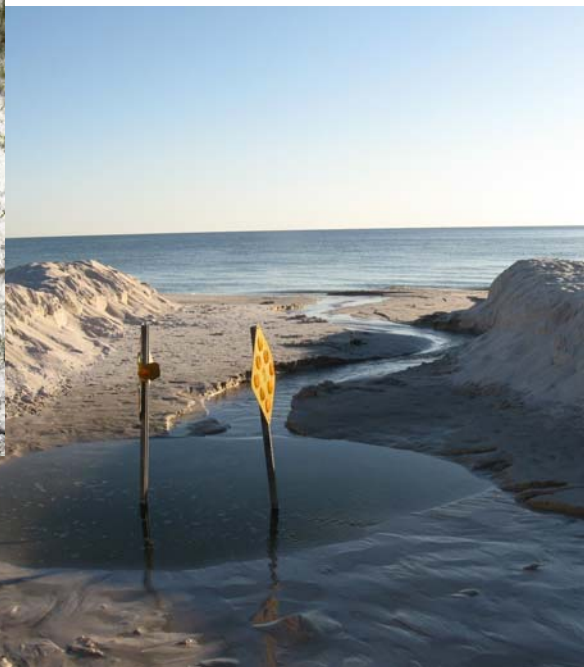
View of the same stormwater pipeline above. Photograph shows the constant stream of water that is unrelated to rain events that flows into the Gulf of Mexico each day. Photographed by Pamela Brown.
