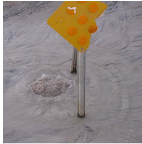
A stormwater pipeline buried under sand on the beach in Panama City Beach. Photographed by Pamela Brown.
