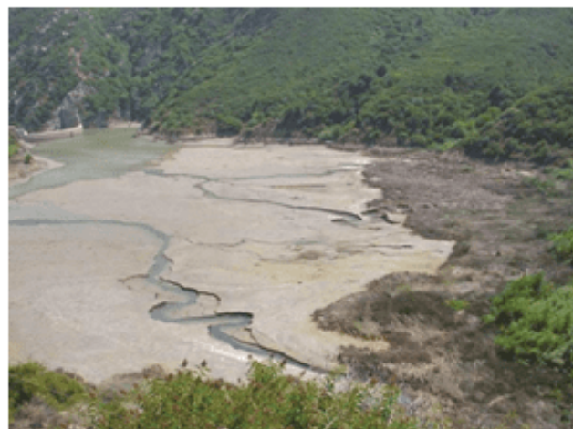
Figure 3-2. Matilija Dam, on the Ventura River Basin, California, is nearly completely filled with sediment. When constructed in 1947, the dam was 190 ft high and impounded a volume of 7,000 ac-ft; by 2015 it was reduced to 400 ac-ft. Photo credit: P. Jenkin.
