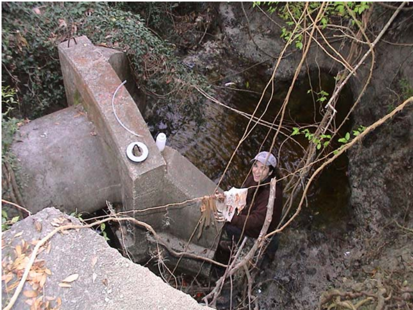
Figure 3-4. Example of a culvert (site 35) with deeply incised creek walls.
