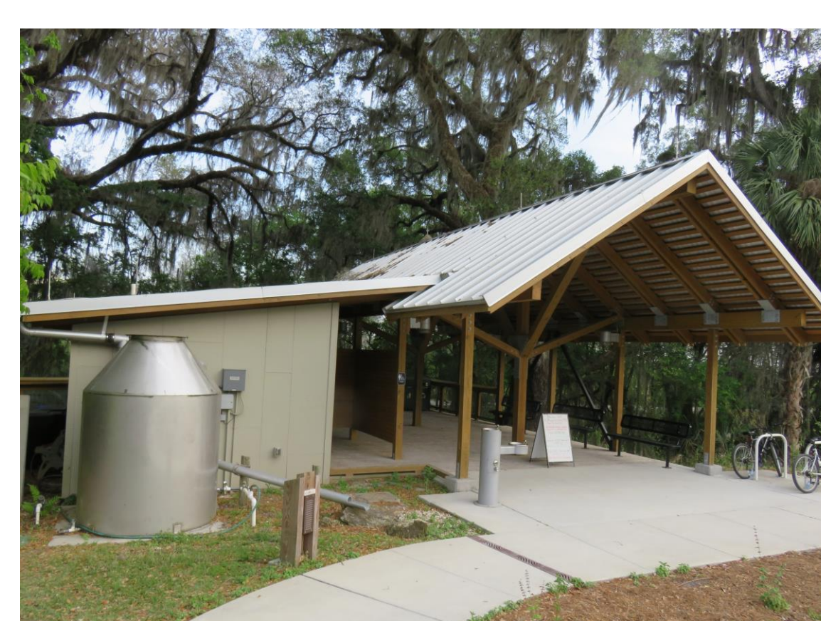
Roof-top rainwater harvester at Gainesville Sweetwater Wetland Park
