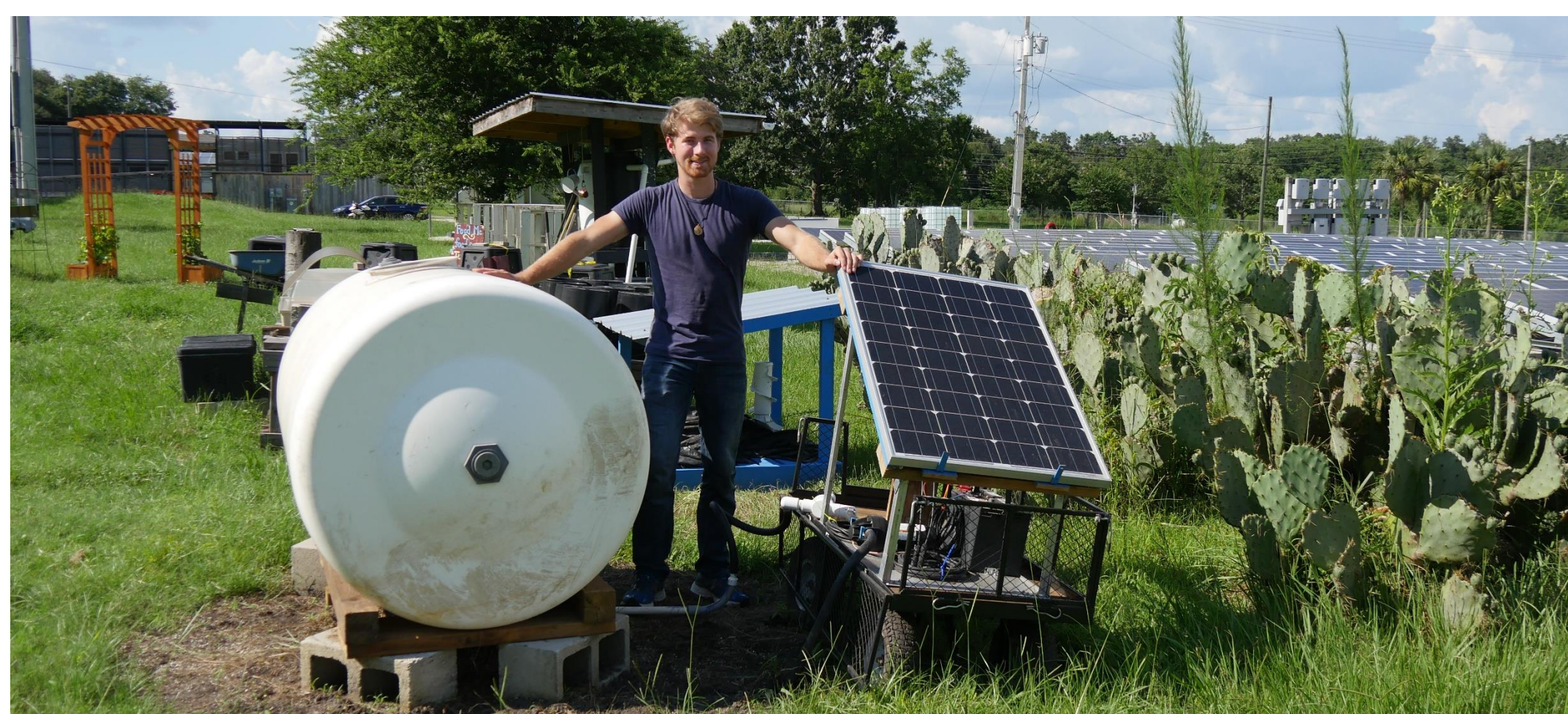
Figure 1. Solar Irrigation Pump attached to rainwater supply.
