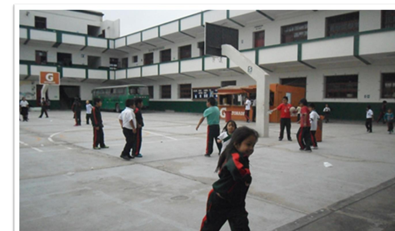
Communal area at Dos de Mayo school
