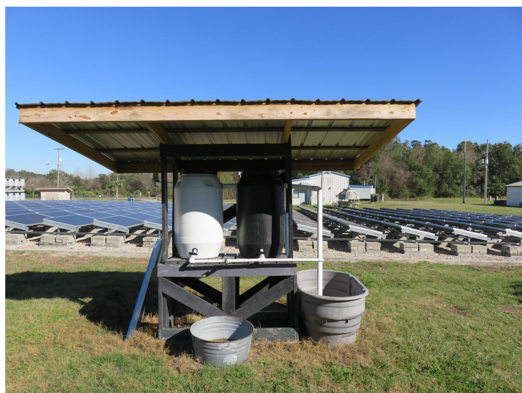
Stand-alone rainwater harvester at the Bioenergy and Sustainable Technology Laboratory
