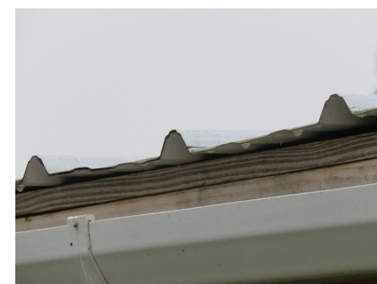
Rain falling into gutter system during 0.25-inch rain event
