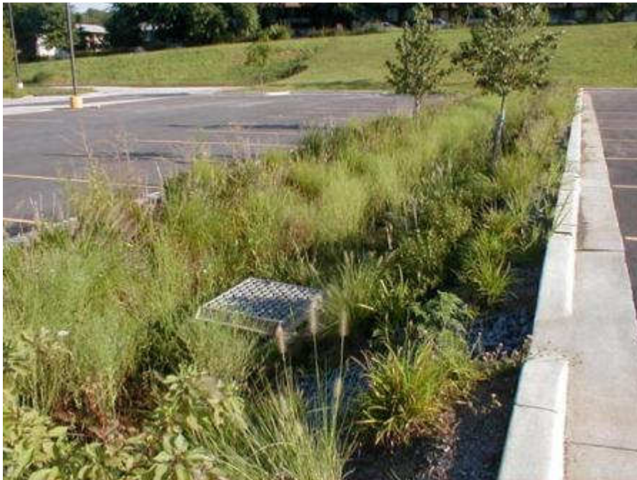
Figure 2: Bioretention facility treating parking lot runoff in Maryland (Davis, 2004)
