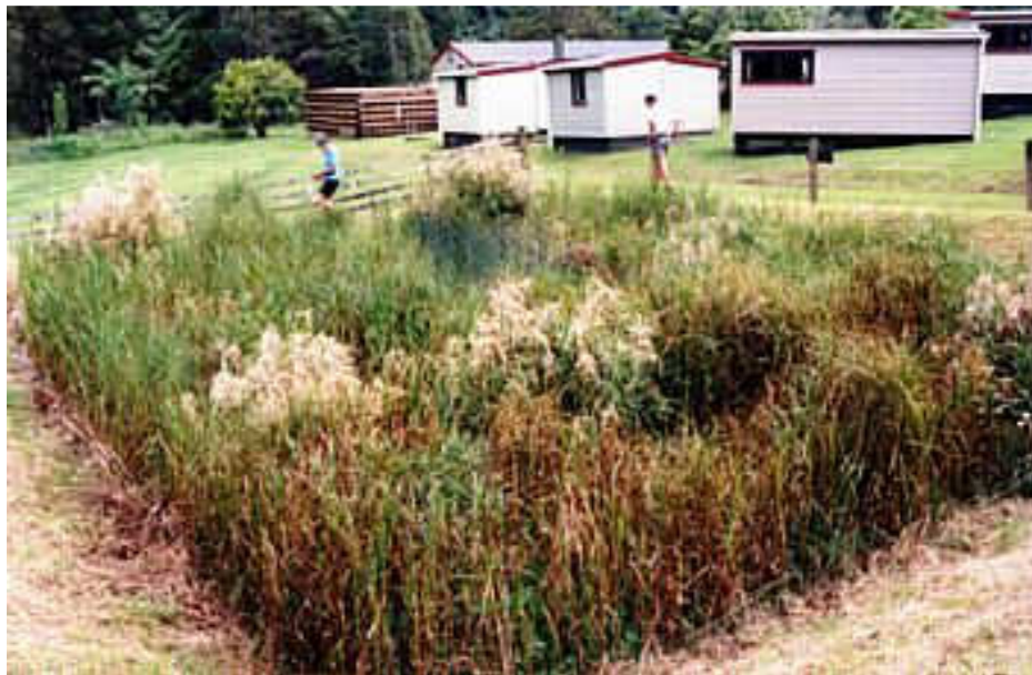
Figure 3: Constructed subsurface flow wetland treating septic tank effluent (Tanner and Sukias, 2002)
